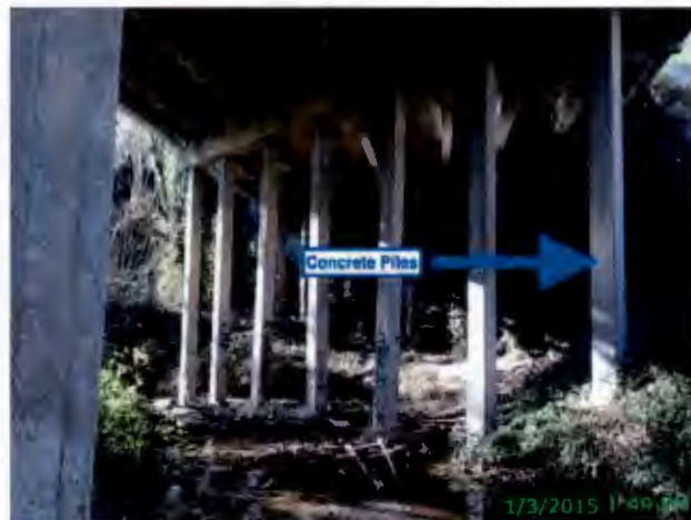
Photos of Traffic Way Bridge
